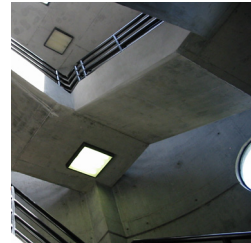
LOOKING UP INSIDE SILO STAIR 03:50 PM 25 JUL 02
