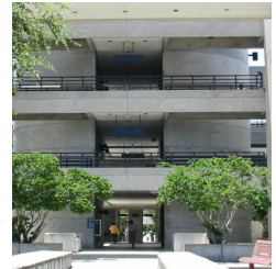
LOOKING WEST AT FRONT ENTRY 02:58 PM 25 JUL 02
